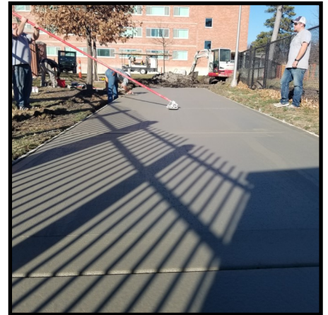
Landscape installing sidewalk between playground and stadium
