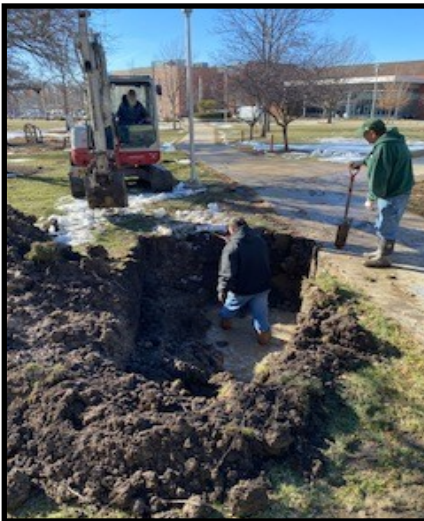
Colden Water Leak Repairs
